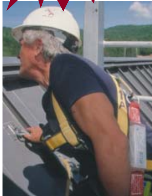
The CSA Learning Centre's one-day Fall Protection workshops provide "hands on" instruction on the proper use of harnesses, shock absorbers and lanyards.
